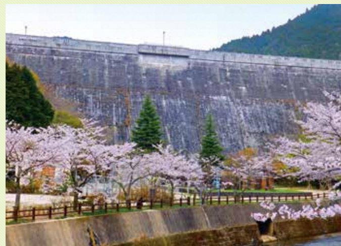
▲Magarifuchi Dam and Dam Park 29 MAP: B-3 The first exclusive water supplying dam in Fukuoka city, built in 1923. This gravity dam, made of concrete with granite stone masonry on the outside was chosen for 100 Modern Water Supply Championship in 1985. Enjoy cherry blossom in spring and colored maple leaves in autumn. The park down stream is good for family outings and pick nicks. ① Magarifuchi, Sawara Ward, Fukuoka
